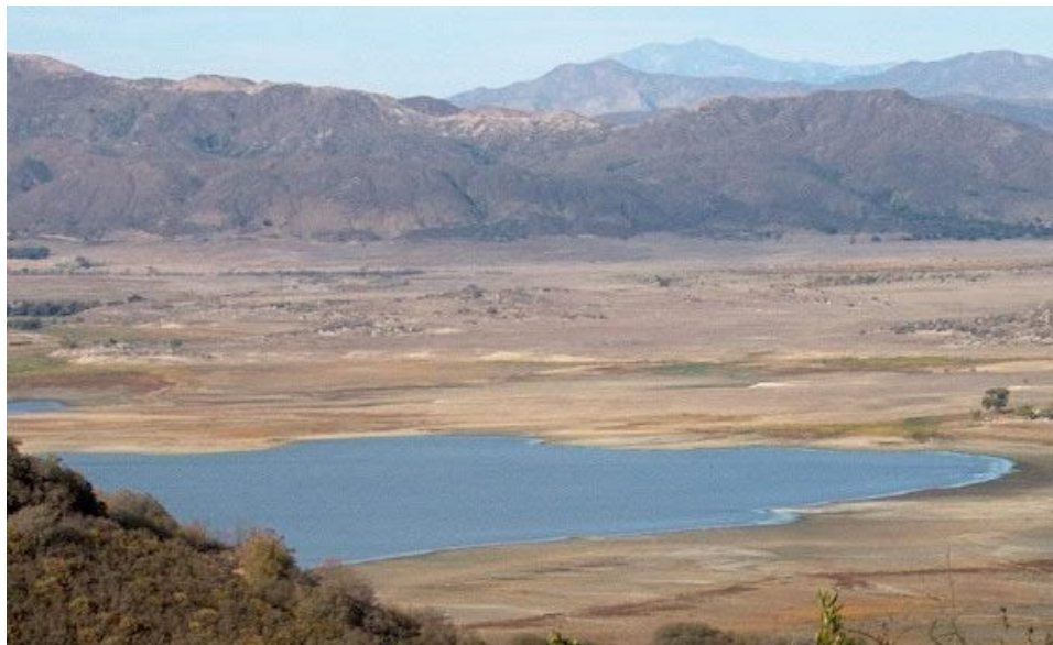
Fig. 5. Lake Henshaw Reservoir in San Diego County has minimal surrounding vegetation and flat topography, reducing the likelihood of direct wildfire damage or indirect post-fire sedimentation.
